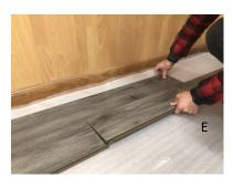
E and F. Finishing rows 1 and 2— continue alternating planks on rows 1 and 2 to avoid misalignment. From row 3 onwards, installation does not require alternating rows. Install one row after the other by starting with angling on the long side, sliding until the short sides are in contact and then locking the short side. As you go, ensure the short sides are securely locked by tapping with your fist, or if need be, a rubber mallet.
