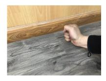
D. Using the drop lock system, drop the short side of the last long plank into the short side of the first laid plank. Slightly tap on the top of the joint of the short side with your fist to secure.
